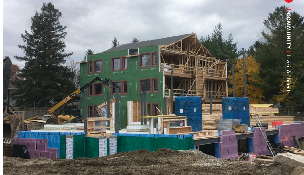
Photos by Greg Leskien, Zon Engineering
